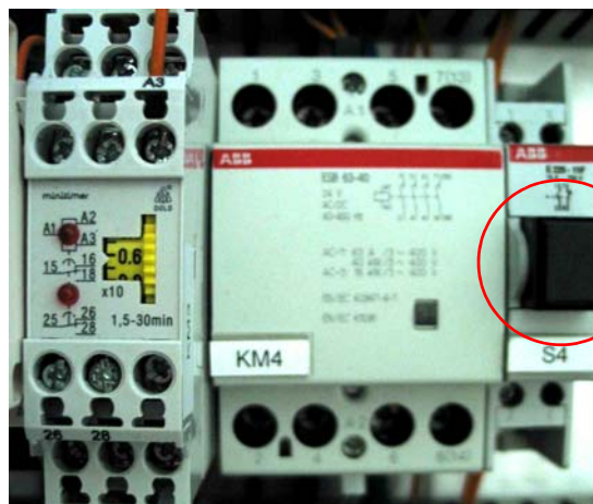
Figure 14.7: Restarting the NMR Console Using the S4 Switch
