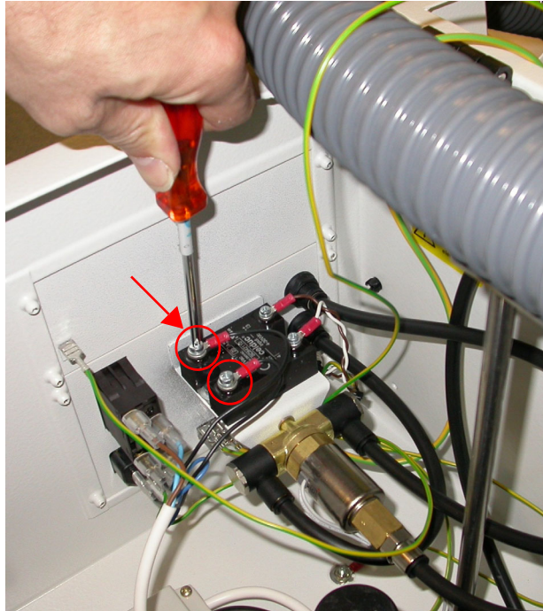
Figure 3.2. Two wires to be disconnect
