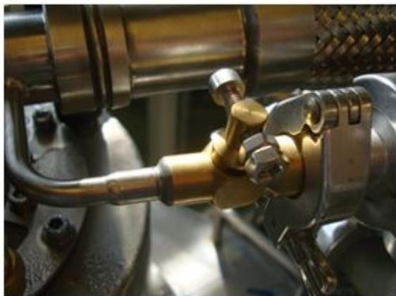
*Figure 8.11: Transfer Line Vacuum Valve Closed*
