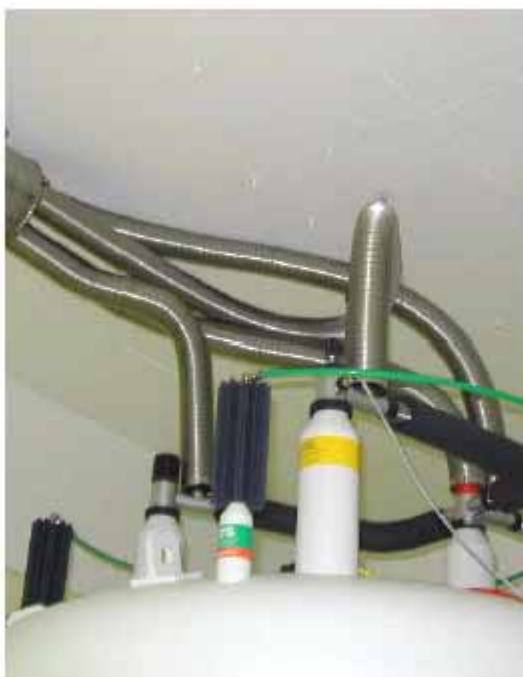
Figure 9.3. Emergency Quench Pipes
