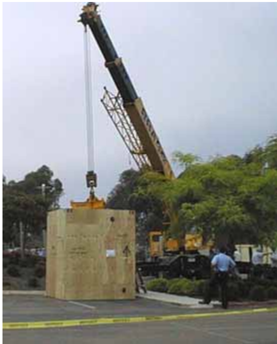
Figure 4.2. Unloading the Magnet Crate and Positioning for Uncrating
