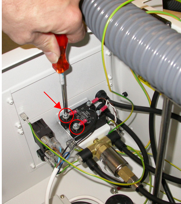
Figure 3.2. Two wires to be disconnect
