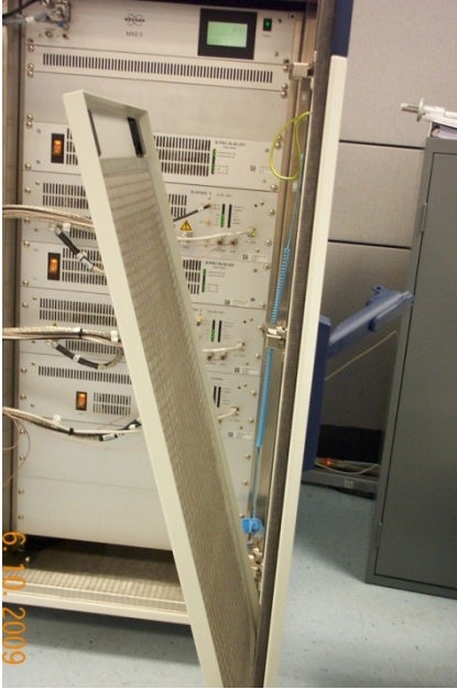
Replacing air filter in door
